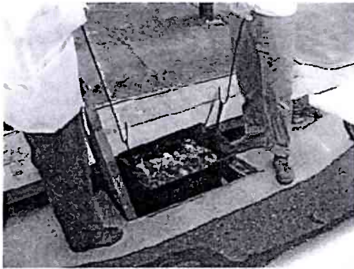
Plate 14 Lift the bag from the stormwater pit
