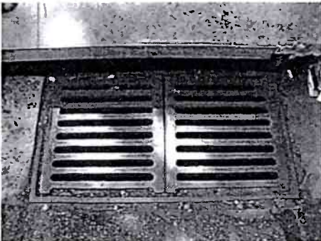
Plate 10 Reinstated non hinged grate
