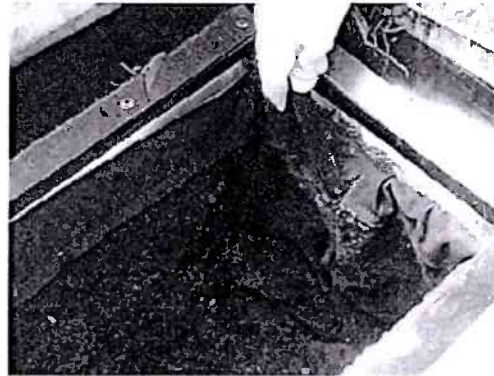
Plate 21 Ensure that the unit is positioned correctly, with the lifting loops on the inside
