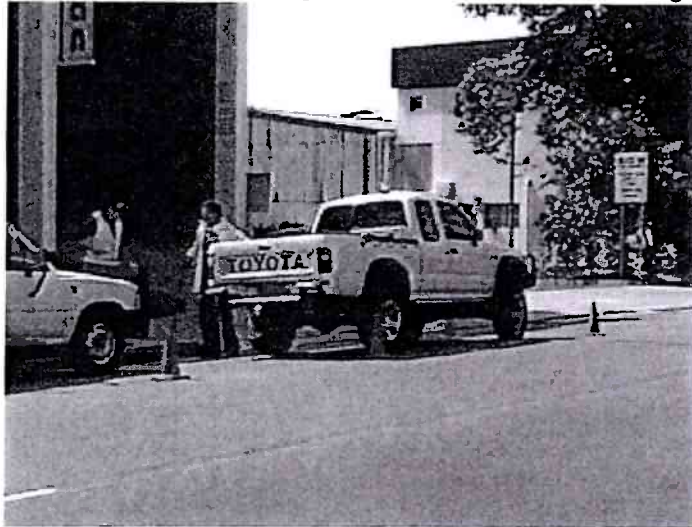
Plate 1 Vehicle positioned near pit, preventing traffic from passing close to the pit.
