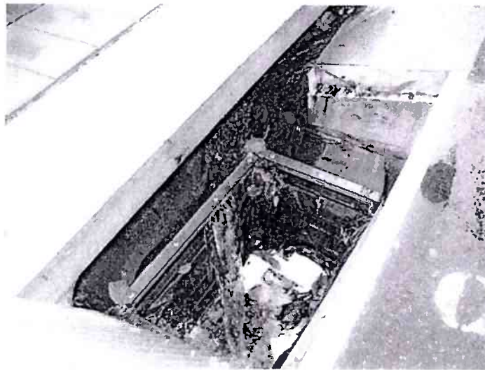
Enviropod filter in service.
