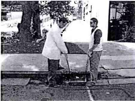
Plate 8 Lift grate and move grate to one side
